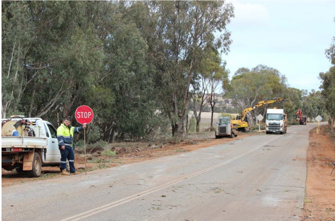
Work on Mogumber – Yarawindah Road
